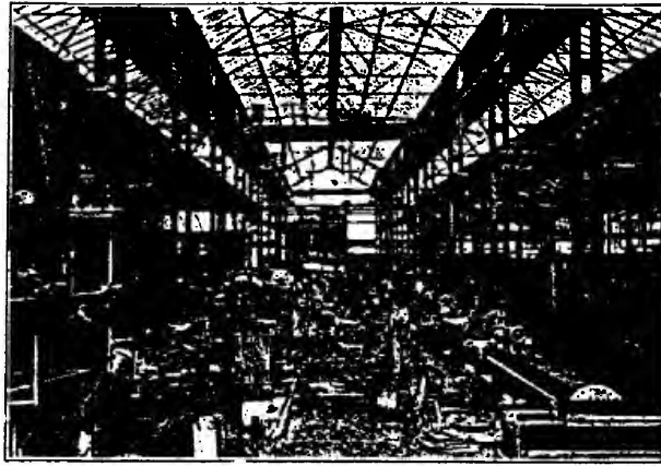
Interior View of Central Workshop
