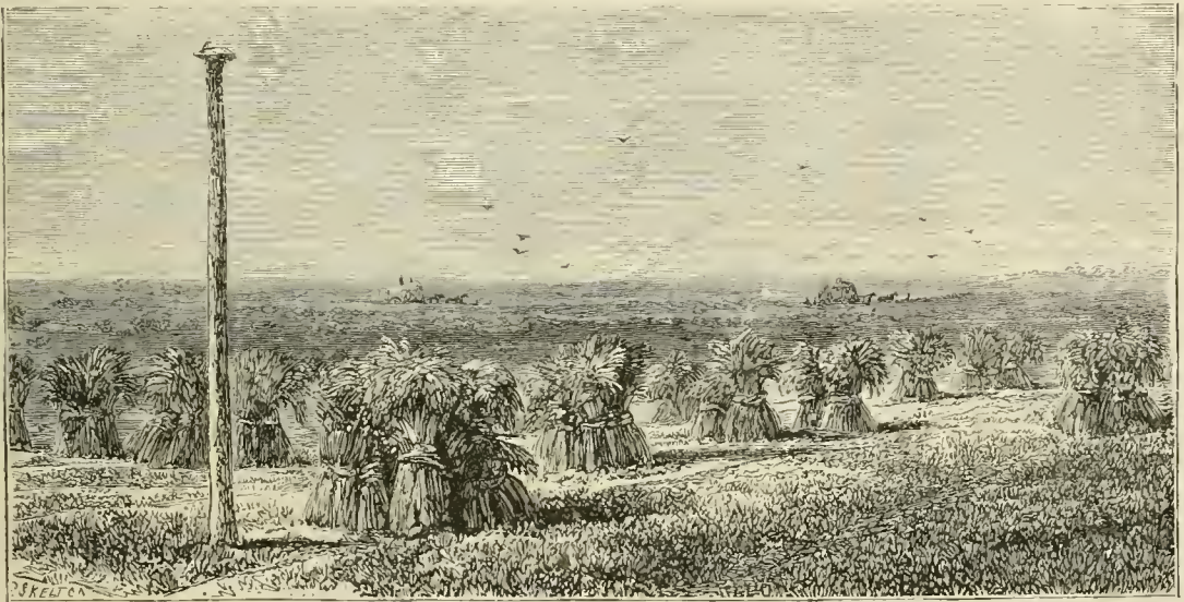
WHITTLESEA MERE AS IT IS. The Iron Post marks the subsidence of the soil (8 ft. 2 in.) since drainage.
