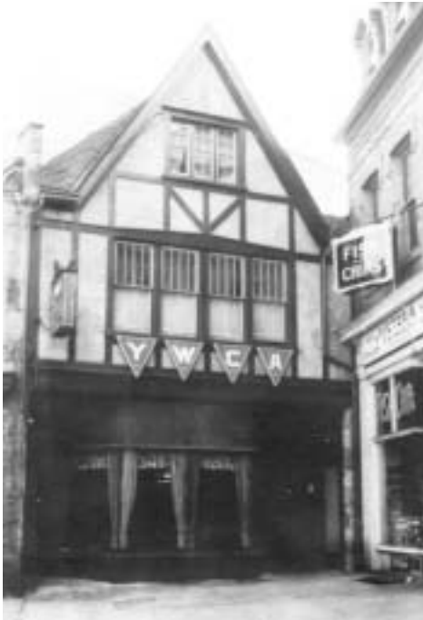
The YM-YWCA has a long history in Guelph and for many decades had a prominent presence in the downtown core. This distinctive YWCA building, ca. 1920, is one of the few historic buildings at St. George's Square that survived the post-war modernization movement.
