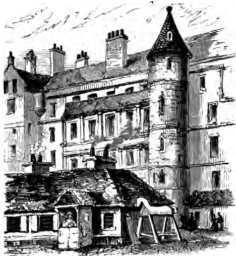
Black Turnpike and Old Guard House.
