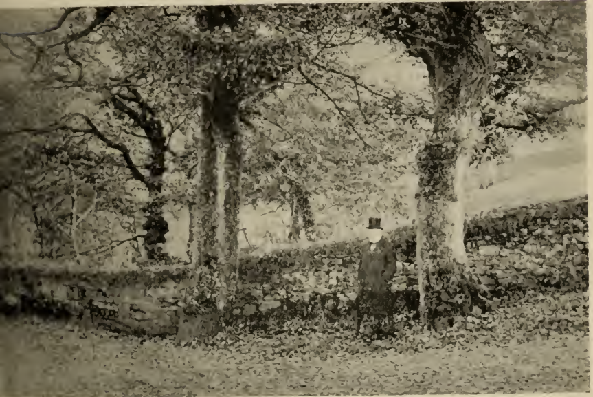
DISRUPTION SCENE AT GILNOCKIE BRIDGE.
