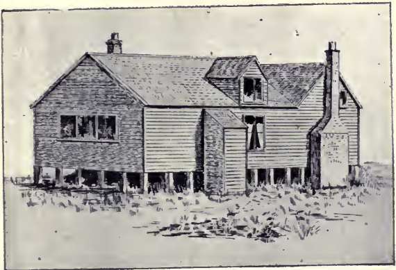
FIRST BOROUGH SCHOOL. SIDE VIEW.
