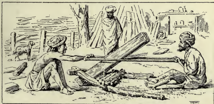
Carpenters at Work.
