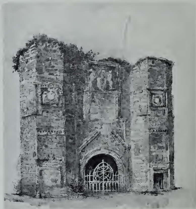
MAR'S LUDGING, MAIN ENTRANCE.
