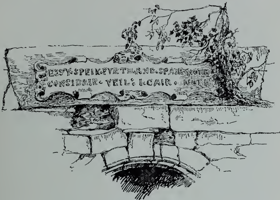
A DOORWAY LINTEL.
