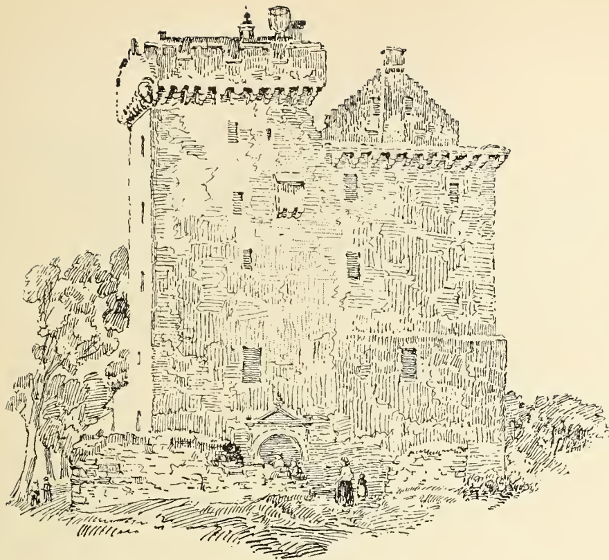
Clackmannan Tower (east view).
