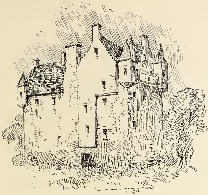
Kilbryde Castle in 1861, prior to repairs.
