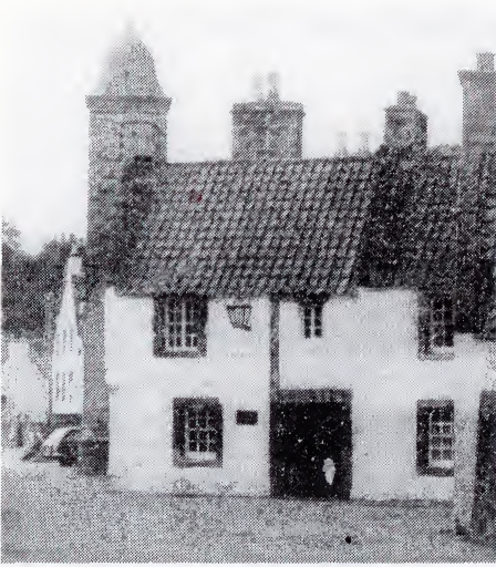
Electricity sub-station, Culross.
