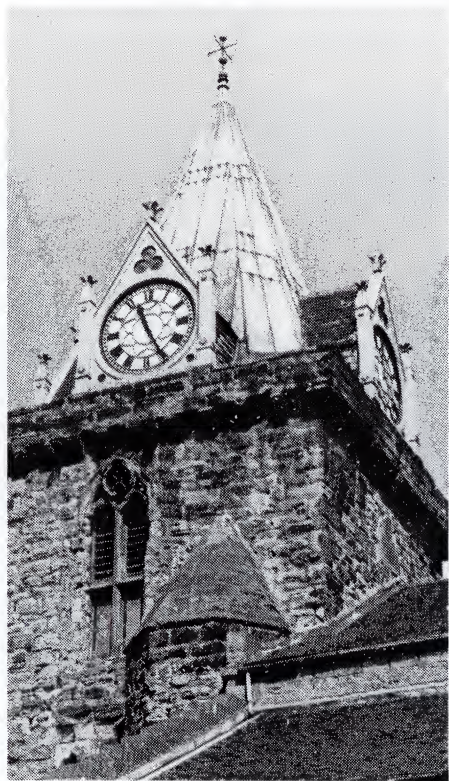
St Peter's Church Tower.
