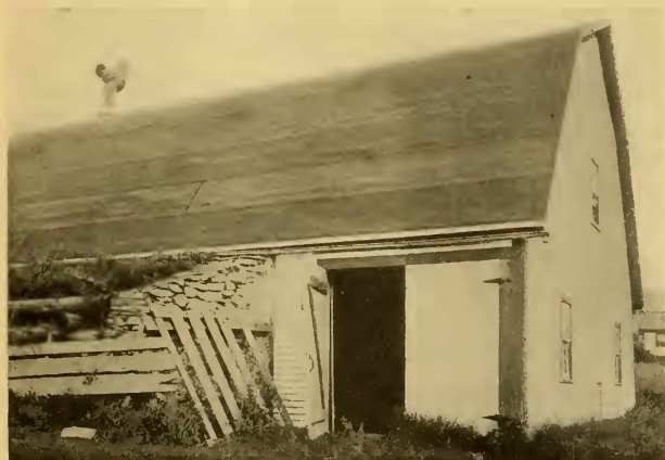
FIG. 131.—Exterior rear view of same house showing driveway entrance located in sole of building at the rear end.
