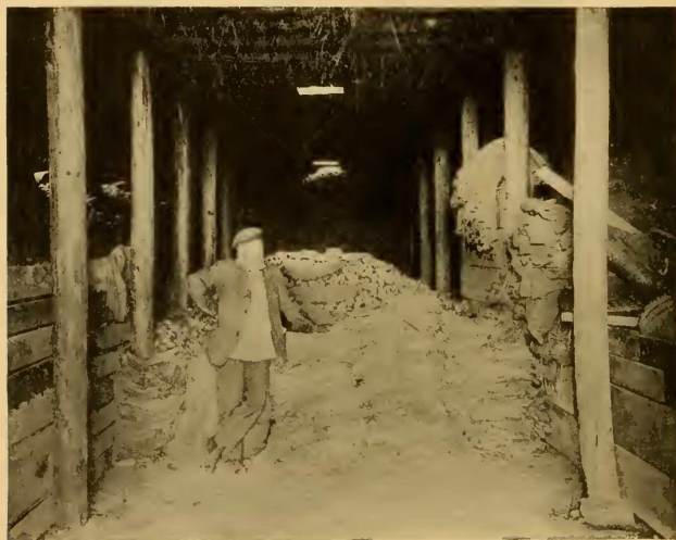
FIG. 128.—Method of filling a storage house in the Greeley district through openings in roof. Driveway partially filled by spooling potatoes through roof openings.
