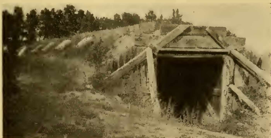
FIG. 115.—One of the cheaper types of partially sunken, earth-covered storage houses with earth retaining walls and side roof openings which may be used for filling the storage space or for ventilation. In the Greeley, Col., district.
