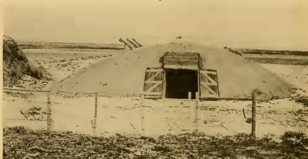
FIG. 120.—A frontal view of the completed potato storage house (Fig. 118) showing driveway entrance and ventilator caps raised on left side.
