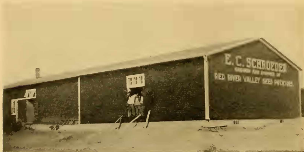
FIG. 124.—A typical Red River Valley potato warehouse with a deep cement-walled basement cellar. Glyndon, Minn.
