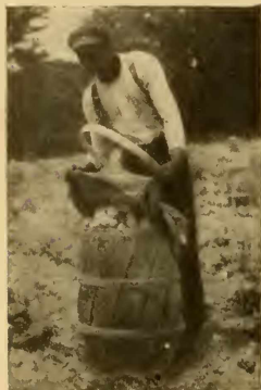
FIG. 99.—A splint barrel being covered. Note light construction of barrel.
