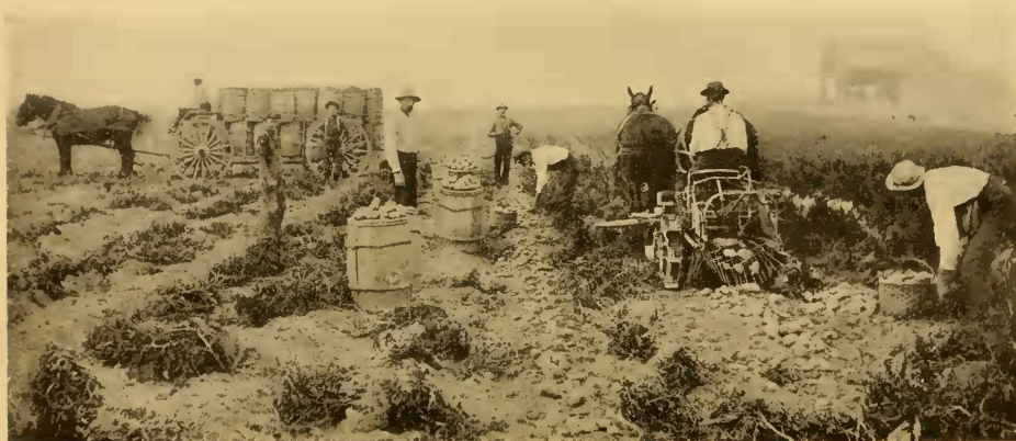
FIG. 84.—The rear rack head in this digger is lowered to a point where the tubers have almost no drop. The picture shows an everyday scene on almost every Aroostook County, Me., farm during September and the early part of October.
