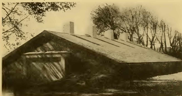
FIG. 123.—Potato storage house with concrete walls, straw and earthen-covered roof plus a superimposed wooden shingle-covered roof. Greeley, Colorado.
