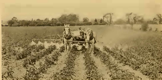
FIG. 197.—Spray outfit hauled by horses, pump operated by a gasoline engine mounted in front of spray tank. Courtesy of Bateman Mfg. Co.
