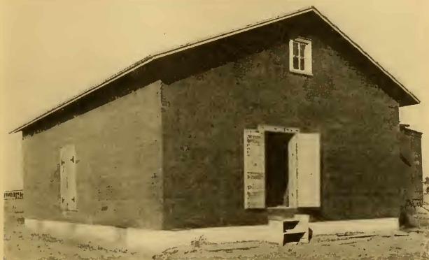
FIG. 129.—A good example of an insulated wooden structure used for the storage of potatoes in some localities in Michigan.
