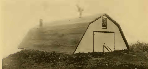
FIG. 130.—Exterior front view of a Maine type of storage house. This particular house is an exception to the general rule in that it is provided with a roof ventilator.
