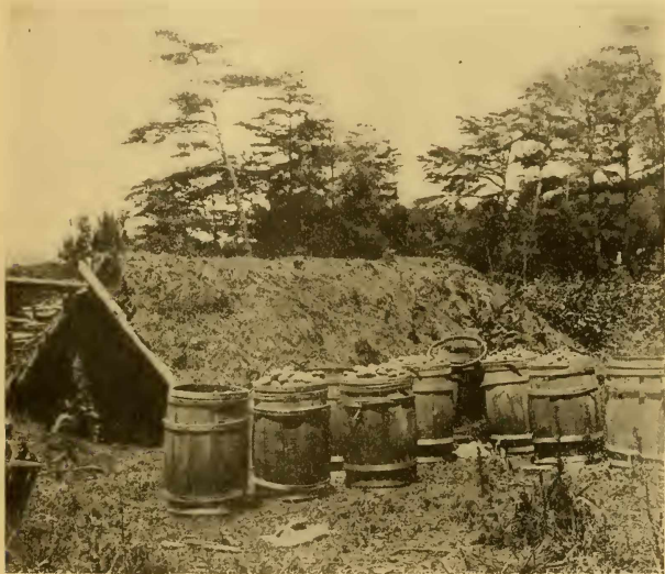
FIG. 117.—A cheaply constructed storage house near Capeville, Va. Roof consists of rough poles resting on the ground and supported by ridge pole at top covered with pine needles. Such a type of storage house would not be suitable where extremely low temperatures prevail.
