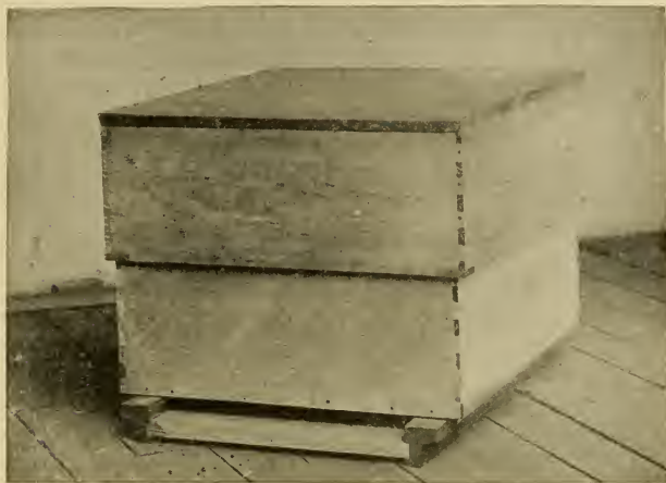
FIG. 113.—Double-walled hive assembled. The double-walled hive with the space between filled with chaff or cork is suited to the conditions of localities where winters are mild.
