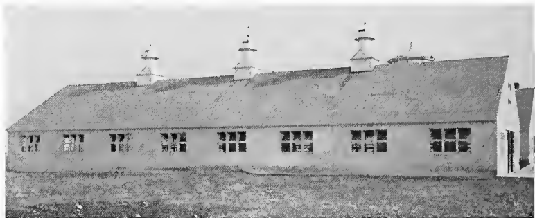
FIG. 85.—A well-lighted dairy barn. Note that top sash of windows fall inward to aid in ventilation. Owned by H. P. Hood and Sons, Boston. (Courtesy of James Mfg. Co.)
