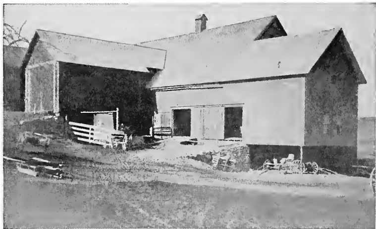
FIG. 61.—A typical Vermont barn. Note team approach on three levels. (Photo by author.)
