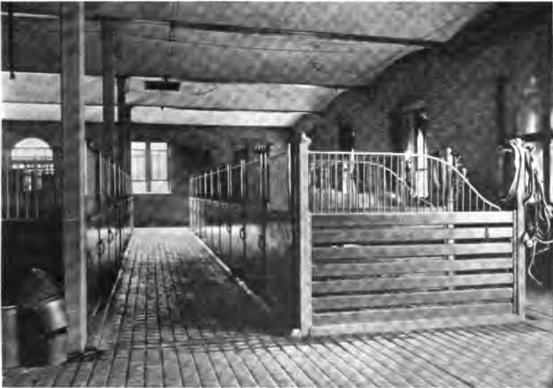
FIG. 131.—A model work horse stable, showing length of stalls, open partitions and front doors, the latter being a convenience for caretakers and obviating the danger of backing heavy horses on slippery floors.
