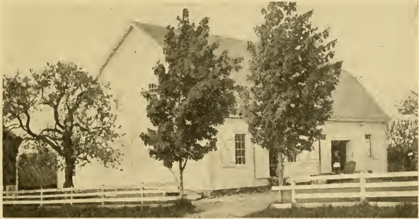
FIG. 120.—A good type of farm storage house. This building will hold about two thousand barrels of apples and has ample room for empty barrels in the loft.
