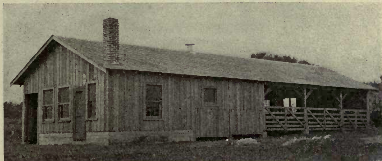
FIG. 166.—An open-shed type of shelter with lambing apartment for cold weather. (From Kentucky Agricultural College.)
