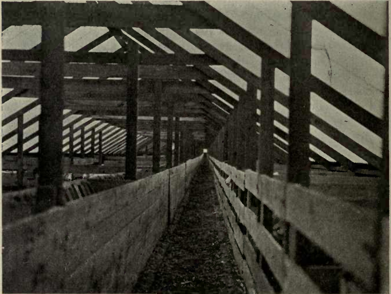
FIG. 231.—A permanent lambing camp consisting of a wooden frame and canvas roof and walls.
