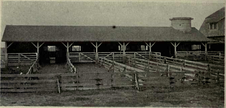
FIG. 237.—Shed, open on one side, University of Illinois; foreground showing fences made of movable panels.
