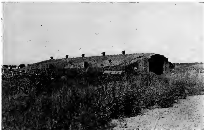
FIG. 183.—Outdoor cellar for storage of potatoes, near Greeley, Colorado.
