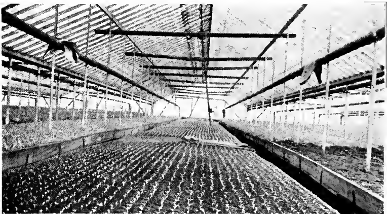
FIG. 189.—Interior view of large range of lettuce houses near Chicago.
