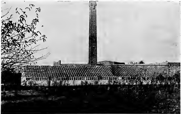
FIG. 33.—A modern greenhouse. The tall smoke stack insures a good draft for the fires.
