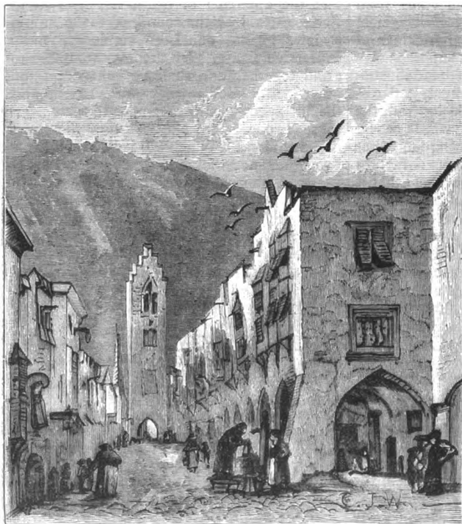
Street and Tower in Sterzing.
