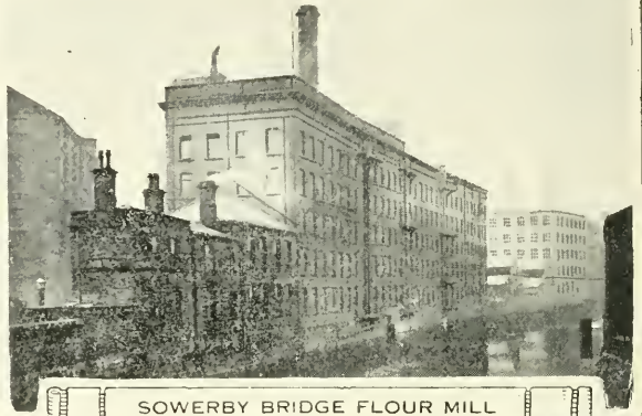
SOWERBY BRIDGE FLOUR MILL
