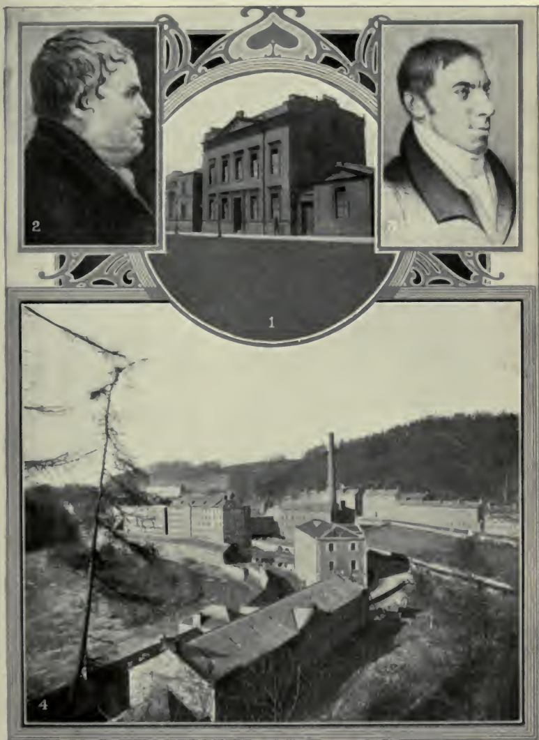
(1) David Dale's House, Glasgow. (2) David Dale.
