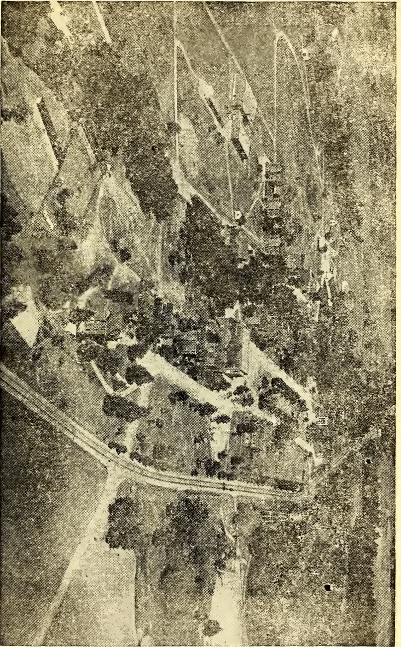
Aerial View of Buildings and Campus.
