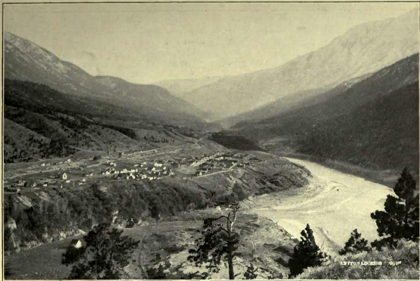
LYTTON, LOOKING SOUTH.
