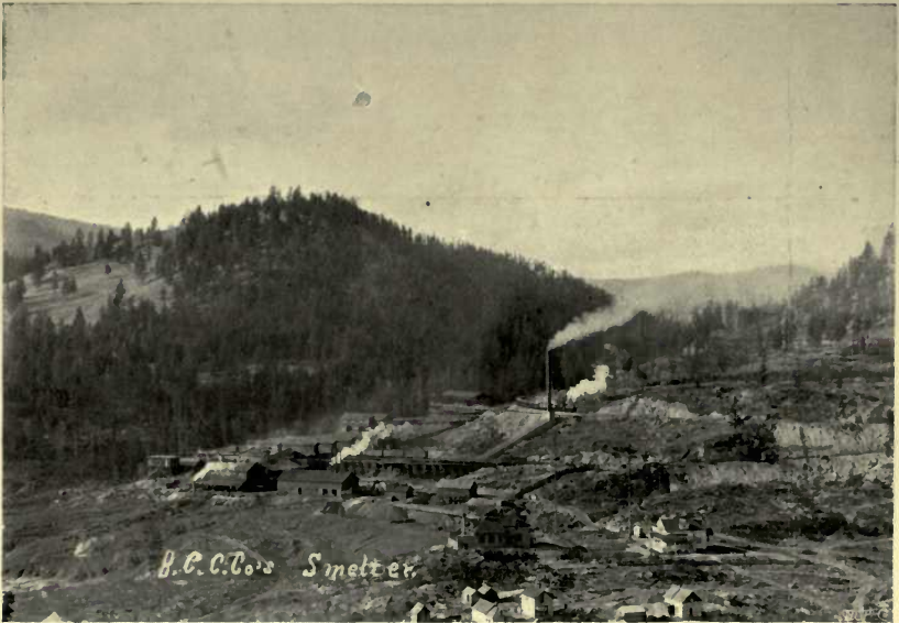
B. C. GOPPER CO.'S SMELTER, GREENWOOD. B. C.
