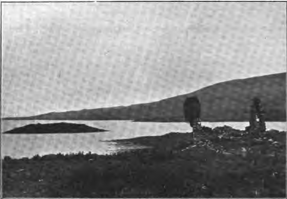
RUINS OF FINLAGGAN CASTLE, ISLAY, AN ANCIENT STRONGHOLD OF THE LORDS OF THE ISLES.
