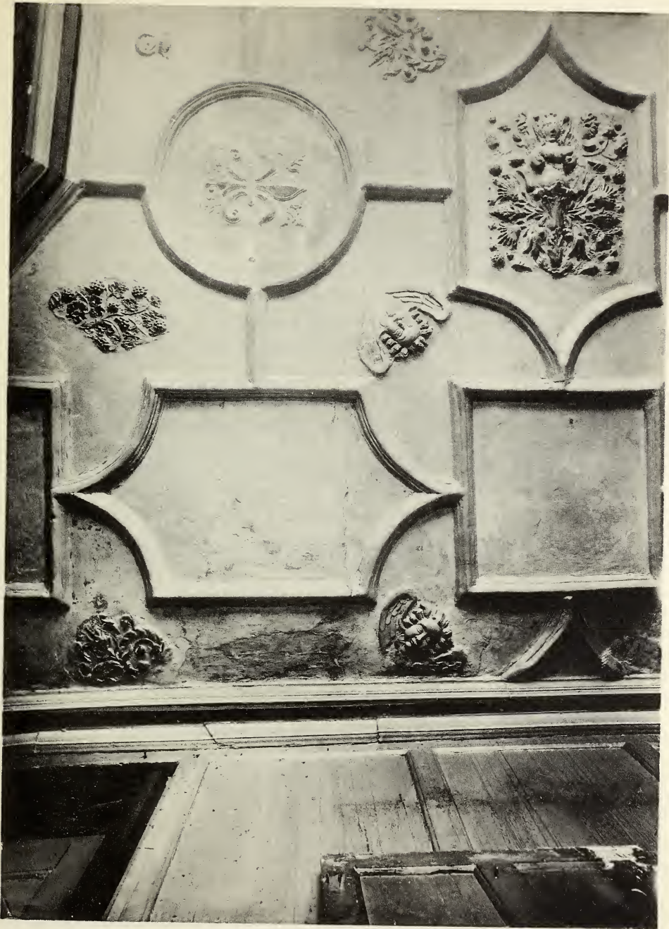
CEILING IN MOUBRAY HOUSE
