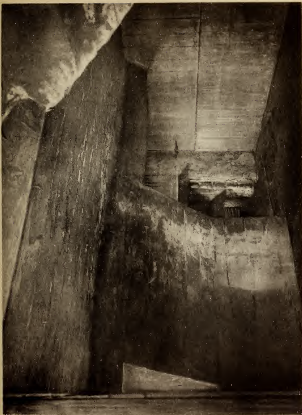
ATTIC ROOM IN COWGATE
