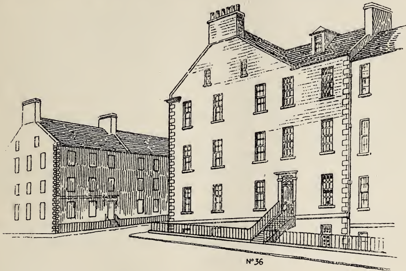
36 Frederick Street as it was in Shelley's time. A new building has been erected on the site.
