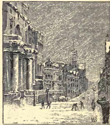
COLLEGE AND SOUTH BRIDGE STREET.
