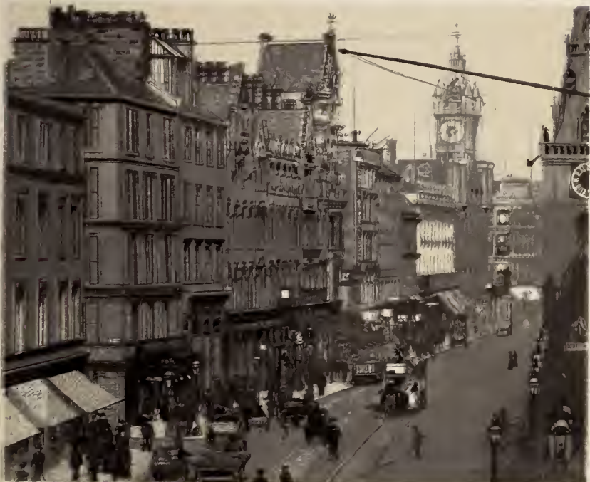
GLASGOW CROSS, TRONGATE
