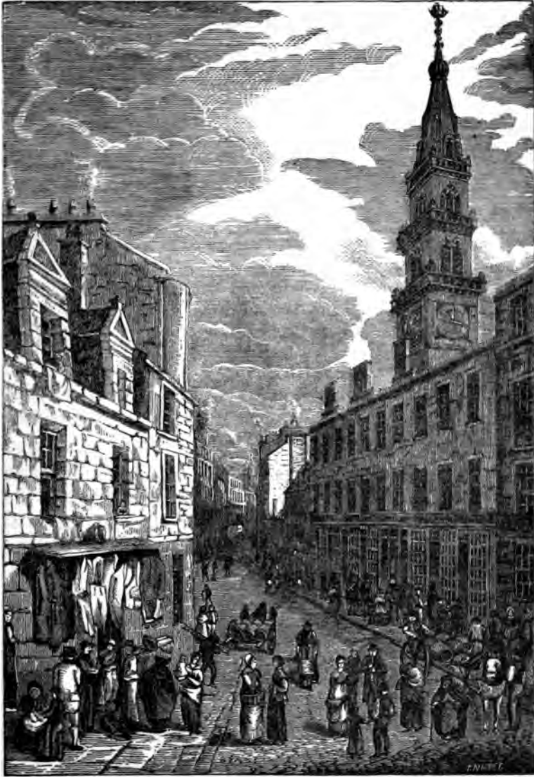
EAST VIEW OF THE BRIDGEGATE FROM STOCKWELL.
