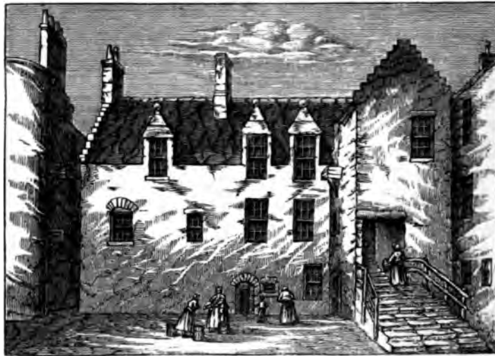
BACK LAND OF HOUSES NO. 157 HIGH STREET.
