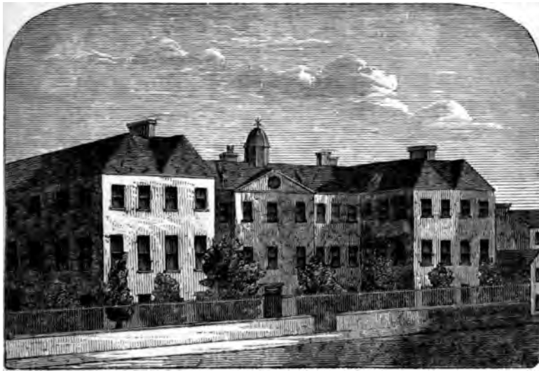
OLD TOWN HOSPITAL., GREAT CLYDE STREET.
