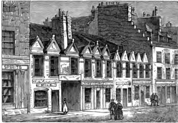
RESIDENCE OF THE CAMPBELLS OF BLYTHSWOOD, BRIDGEGATE.
