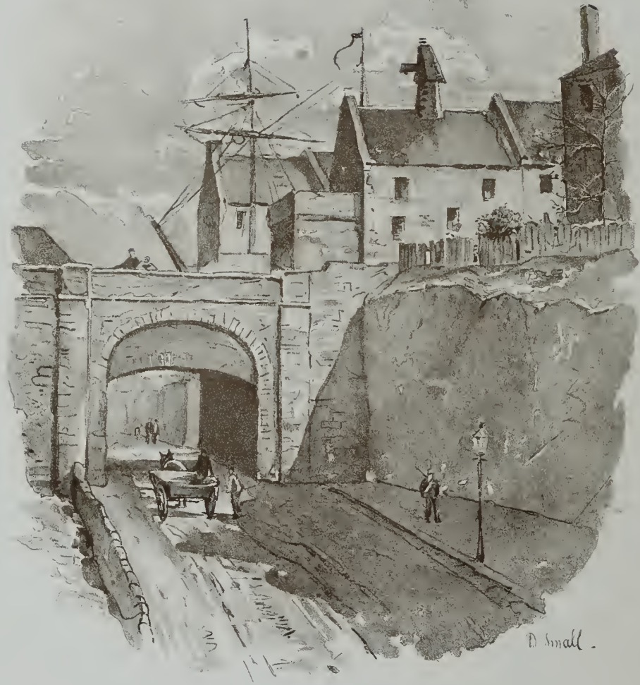
CANAL BRIDGE, BLACK QUARRY. — 1879.
