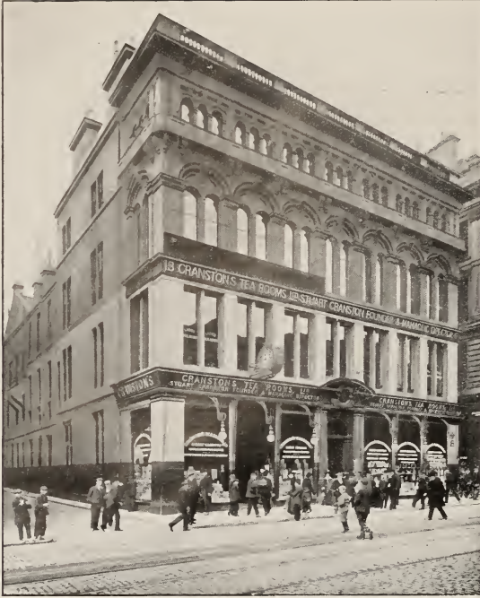
Exterior of 13 Renfield Street.
