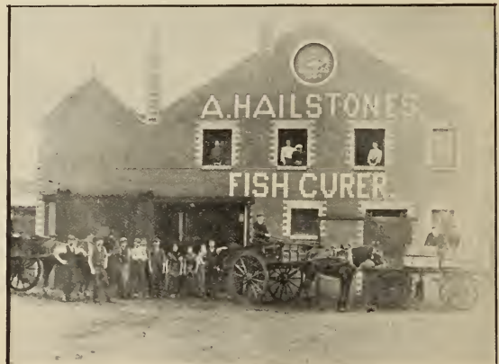
VIEW OF CURING WORKS, GOVAN.
