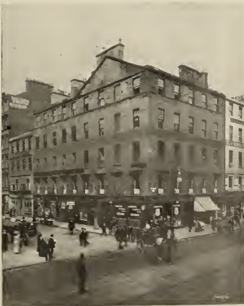
76 Argyll Street and 2 Queen Street. "The old original corner," foot of Queen Street.
