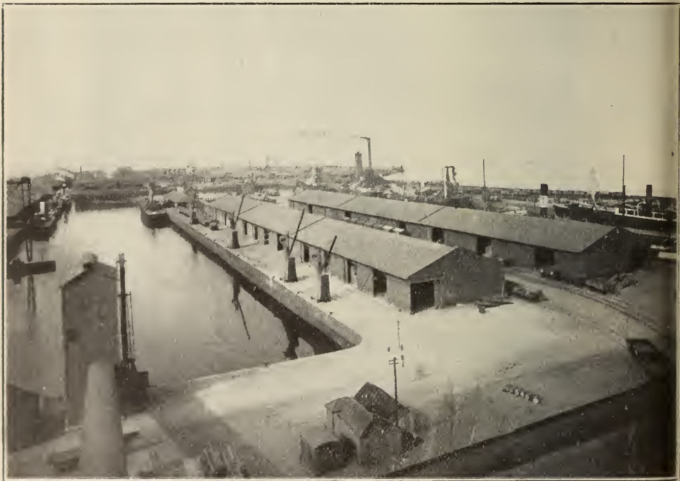
View from Grain Elevator
