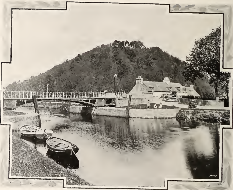
THE CANAL BRIDGE.
