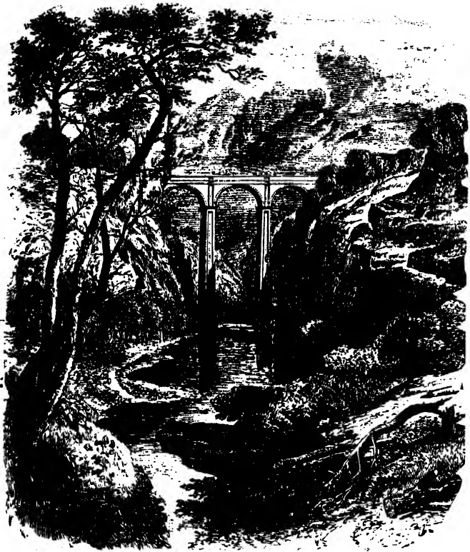
CARTLAND CRAGS BRIDGE.
