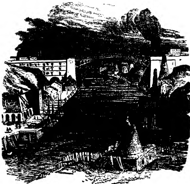
WEAR BRIDGE, AT SUNDERLAND. [By Percival Skelton.]
