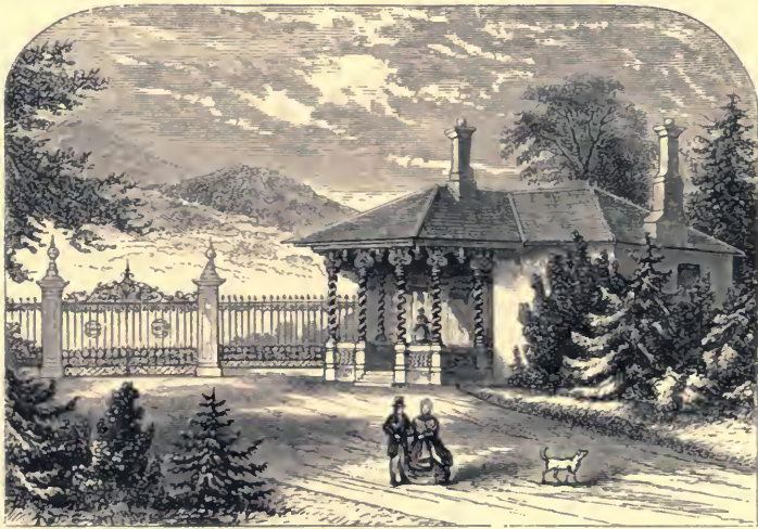
Fig. 55.—Lodge and Entrance, Glenormiston.
