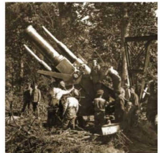
ABOVE: A British 15-inch howitzer being prepared for action. Its high-explosive shell weighed 1,400 pounds, and it had a range of nearly 11,000 yards
