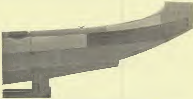
FIG. 49. HULL PLATING BEFORE COMPLETION OF REPAIRS
