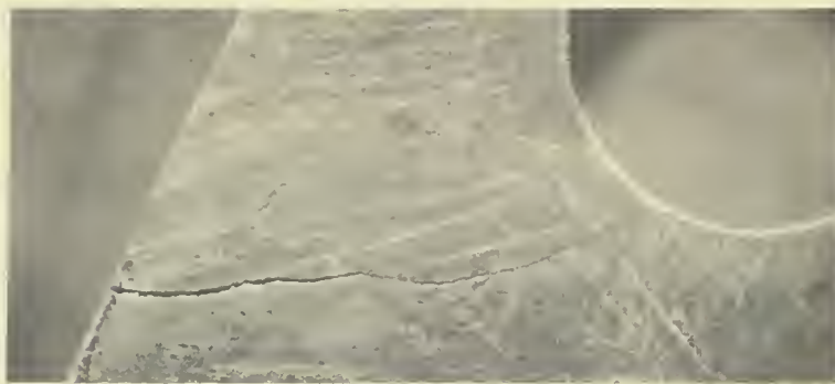
FIG. 14. STAINLESS STEEL - INTERCRYSTALLINE CORROSION
