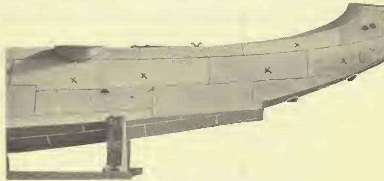
FIG. 50. SHOWING PLATING OF HULL AFTER REPAIRS
