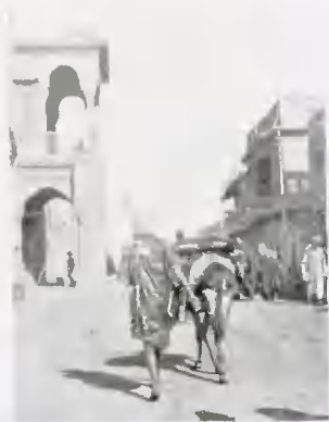
ENTRANCE TO ASHAR BARRACKS.
