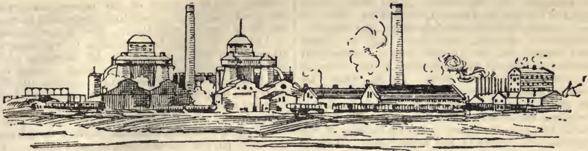
ILLINOIS STEEL COMPANY'S WORKS, NORTH PORTION.
