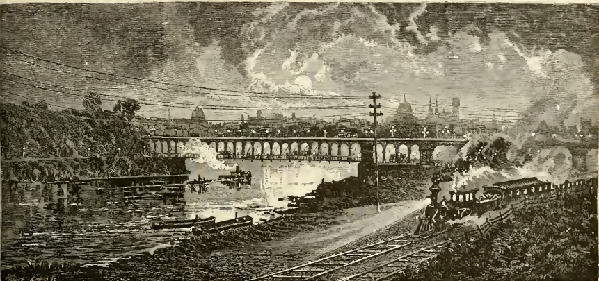
ALLOWHILL STREET BRIDGE, FAIRMOUNT.
