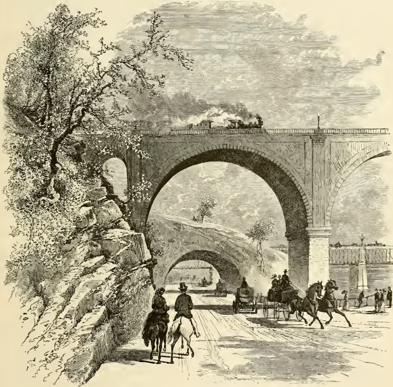
BRIDGE AND TUNNEL IN FAIRMOUNT PARK.
