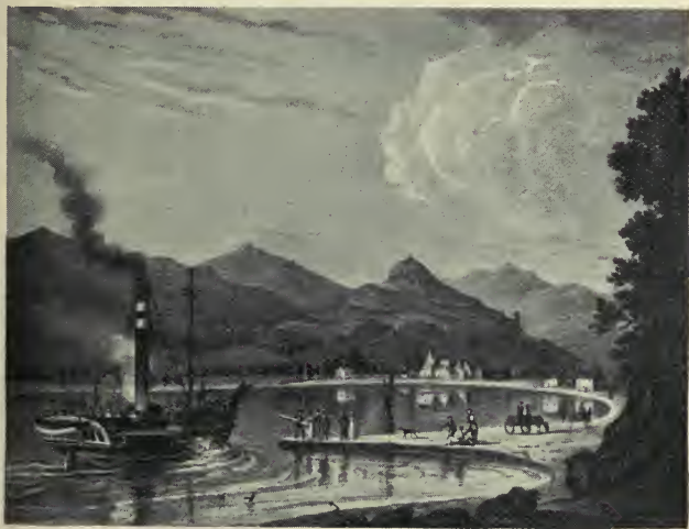
AT LOCH GOIL JETTY
