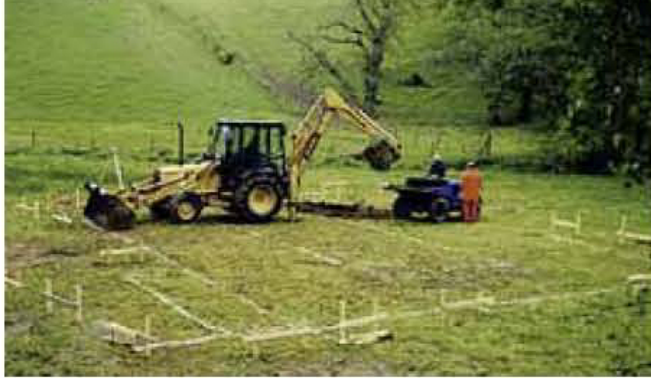
Marking out and starting foundations
