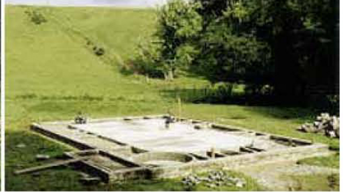
Marking out and starting foundations
