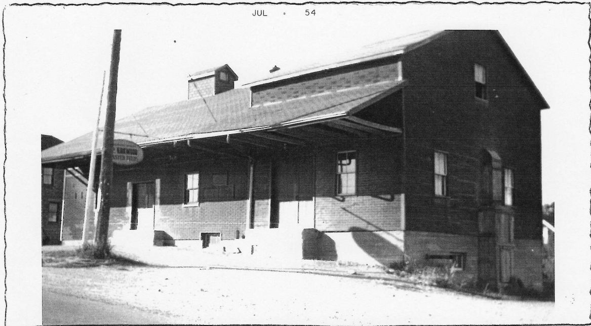
J.P. Kirkwood Grist Mill and Seed Cleaning plant still running today.
