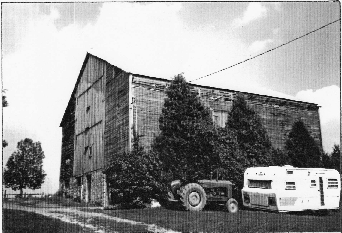
Modern tractor in front of barn at Jim's parents' home place, 10th line, August 1990. On the end, notice how the old barn was enlarged by being split in two and a whole new centre section added.
