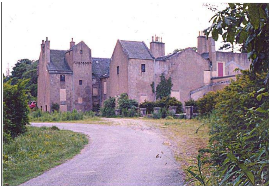
Durriss House: North-East Civil Defence Group Control Centre
