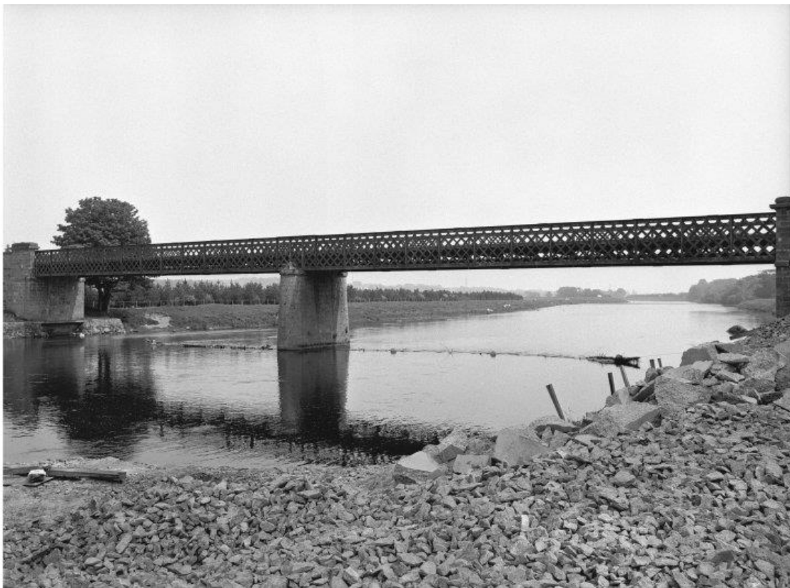
Durris Bridge (Built 1862, replaced 1977)
