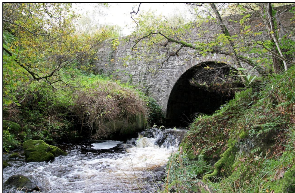
Balladrum Bridge, Durris
