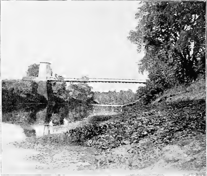
THE FIRST SUSPENSION BRIDGE IN INDIA, BUILT OVER THE BEAS RIVER BY COLONEL DUNCAN PRESGRAVE.
