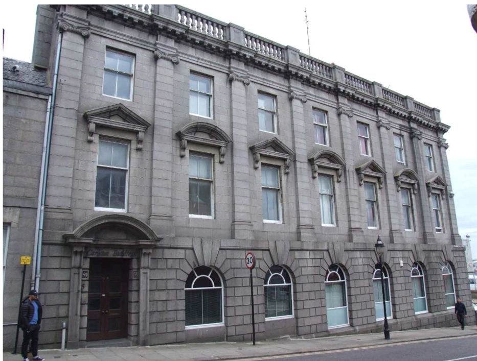
No. 59 Marischal Street, Aberdeen, former offices of William Leslie & Co.
