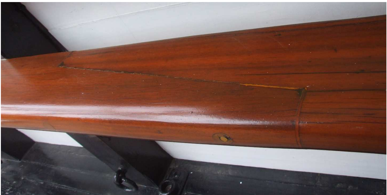
Scarphed connection on the bulwark of RRS ' Discovery '. (S. Bruce).
