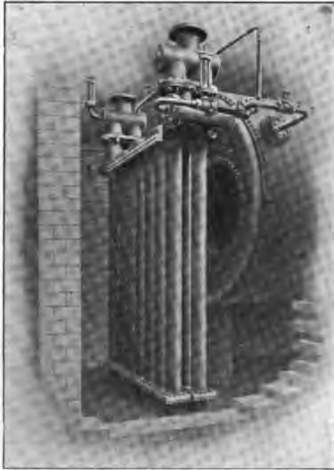
Fig. 47.—Sixteen Pipe Superheater.
