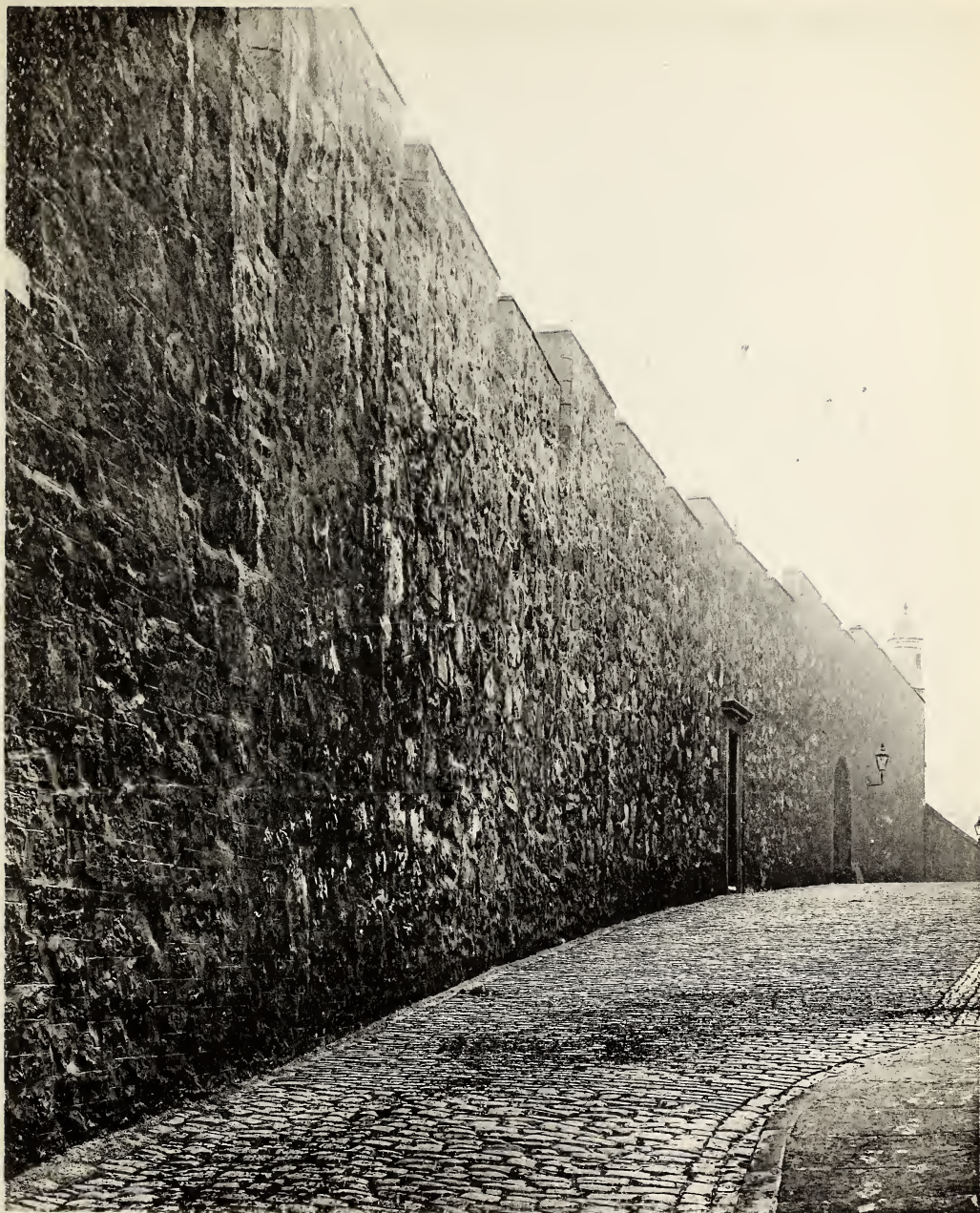
THE VENNEL. THE THIRD CITY WALL (TELFER'S).
