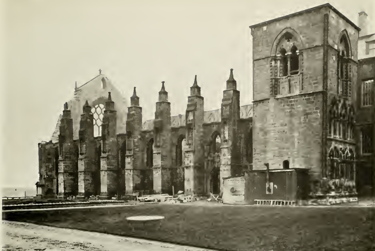
(1) NORTHERN FRONT, WITH THE BUTTRESSES ERECTED BY ABBOT CRAWFORD, 1460-1483
