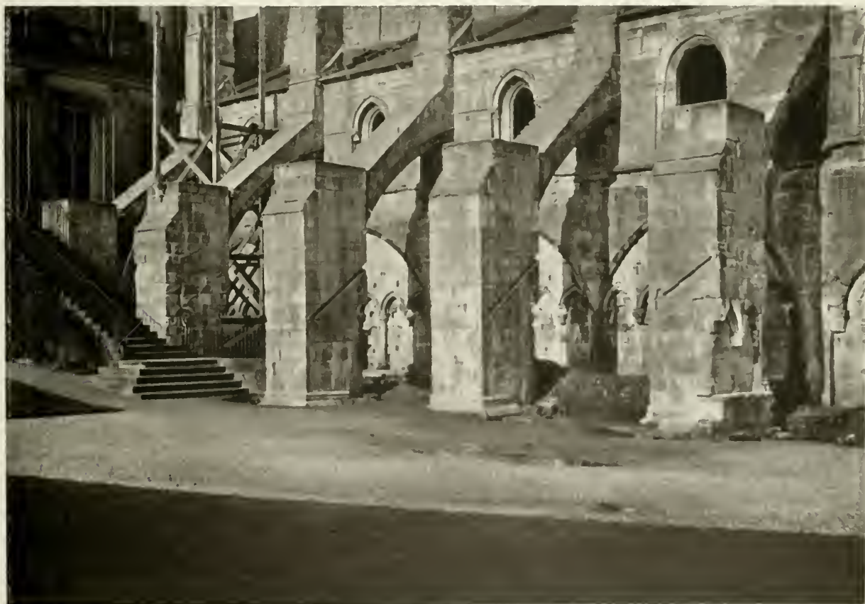
(2) SOUTHERN FRONT, WITH THE BUTTRESSES AND FLYING ARCHES ERECTED BY ABBOT CRAWFORD, 1460-1483
