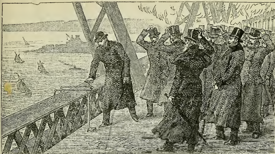
THE OPENING OF THE FORTH BRIDGE.
